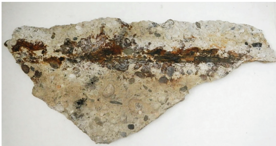
FIGURE 5 Close-up photograph of the rebar inside core sample with thickness loss shown at the top. The corrosion risk was captured early on. Corrosion mitigation and cathodic protection prevented catastrophic failure in a 100-year-old building.
